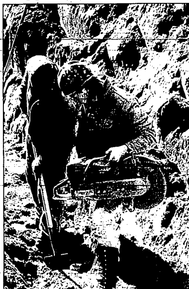
Construction workers Gary Pawson, with saw, and Mark Nevada of Walton Inc. replace deteriorating clay sewer pipes at G Street and 8th Street in Rupert.
