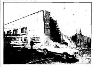
Workers move a trailer next to a collapsed warehouse in Klamath Falls, Ore. Building inspectors say the brick warehouse collapsed Monday because of a series of earthquakes in the area since September. About 20 cars were in the warehouse when it collapsed.
