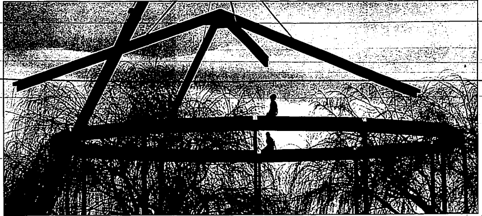
Working on the construction of the new planetarium at CSI, Garon Kelly, front, looks to the sky as a crane lowers a steel structure for the upper dome of the addition to Herrett Museum. Kelly and Tory Jasper were helping guide the piece into place on Wednesday. The $3.6 million project, which includes a 150-seat state-of-the-art planetarium, will add 10,560 square feet of space to the existing museum. It is scheduled to be completed by October.
