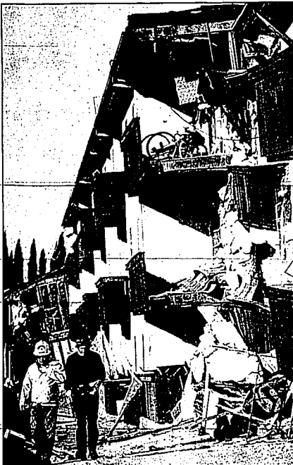
Relief workers examine the Northridge Meadows Apartments soon after the earthquake struck, heavily damaging the complex in Los Angeles, Jan. 17, 1994. The quake, which registered 6.6 on the Richter Scale, killed 16 people in the building.
