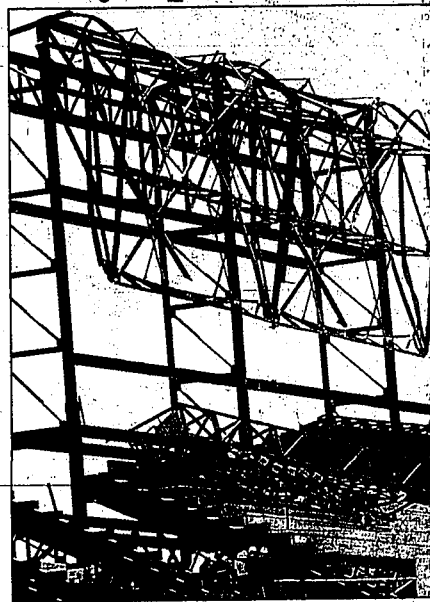
City and Olympic officials are dwarfed by a bank of lights that collapsed at the 1996 Summer Olympic Stadium construction site Monday. One construction worker was killed in the accident and two were injured.
