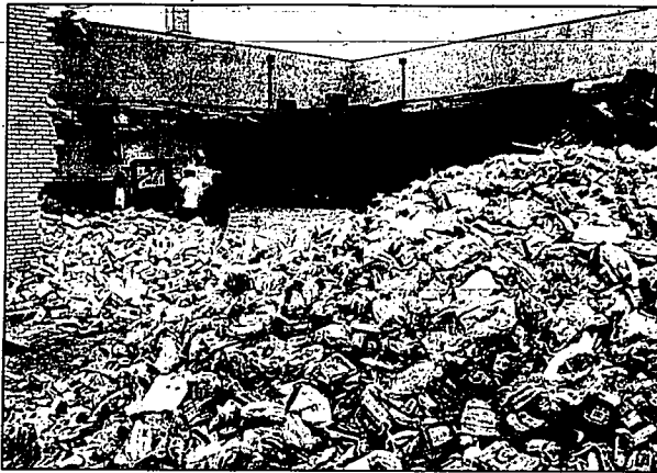
A pile of damaged bread products sits outside a bakery Sunday in Dallas. The bakery's roof collapsed after a storm last week.
