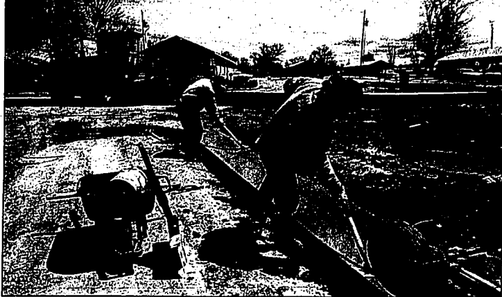
Concrete workers Oscar Gonzalez, right, and Mike Smith shape a new curb and gutter section of the $228,016 El Milagro street project on Friday.
