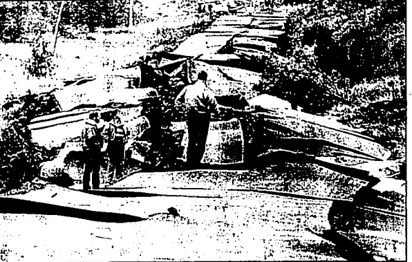
Curious residents examine damage to the McDowell Creek Road near Manhattan, Kan., Wednesday after floods and wet ground caused it to break up. The road slipped 18 feet down a hillside in some places.
