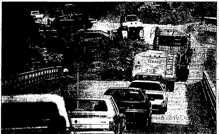
Motorists move slowly around crews using heavy equipment to rip up and haul away part of Clear Lake Grade. Below, the new grade is taking shape as a large wedge of the canyon wall gave way for the road.
