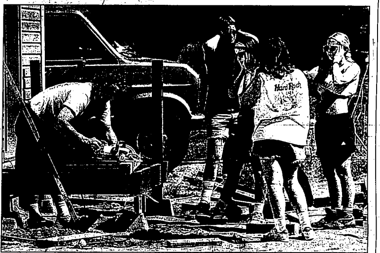
'Building decks is our forte,' said Lyle Ford of Arlington, Wash., referring to his crew of teenaged girl volunteers from Christ Lutheran Church. 'We are the deck-masters.' Even so, it was obvious that Ford's co-workers were not accustomed to loud power tools.
