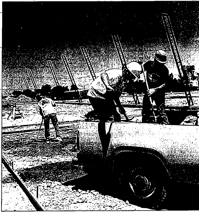
Jeff Slepert, from left, Paul Arrington and Sergio Carrillo level the ground for a concrete floor at the new Lamb-Weston Inc. potato storage building under construction in Twin Falls.
