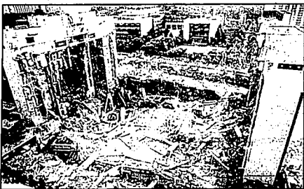
Wrecked walls flank the rubble of the five-story Sampoong Department Store in Seoul that collapsed June 29.
