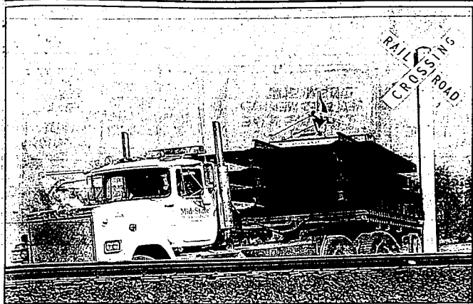
A truck loaded with replacement railroad ties leaves Hyder, Ariz., Wednesday and heads seven miles away to the area of track where an Amtrak train derailed Monday. Repair efforts have already begun as the FBI continues to investigate the scene.
