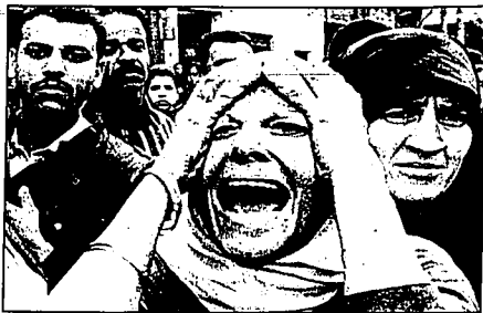
A woman watches as a bulldozer rips into her apartment building Wednesday in Cairo. The building, first damaged in a 1992 earthquake, was irreparably damaged after Wednesday's quake.
