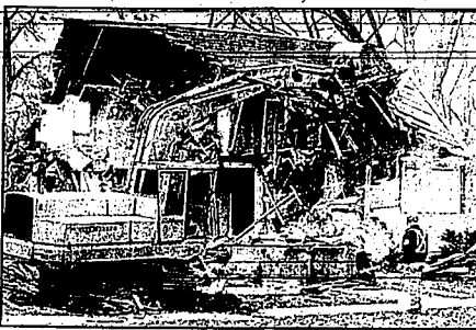
Demolition workers raze Paul Bernardo's house in St. Catharines, Ontario, Canada, on Tuesday in a ritual intended to help this city move beyond the trauma inflicted by Bernardo.
