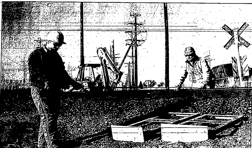
Paul Rodgers of S.S. Electric and Eric Carrington of J.D. Dayley and Sons Install a signal maintainer for a future crossing gate in Hoyburn on Friday.
