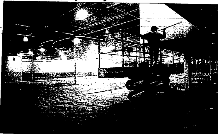
Jerome painter John Hansen works on the vast interior of the Fred Meyer store under construction on Blue Lakes Boulevard in Twin Falls.
