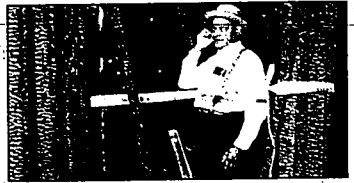
Rev. Chester Thomas, the pastor, surveys fire damage to the New Lighthouse Prayer Church in Greenville, Texas.
