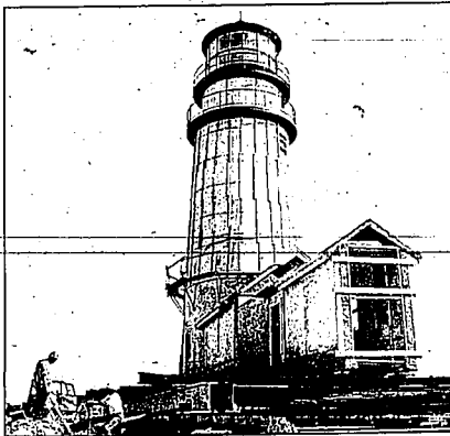
With the Highland Lighthouse lifted off its foundation, helper Jerry Matyko, left, and his worker Michael Landon connect the last hydraulic unit to a steel brace under the Cape Cod lighthouse in North Truro, Mass.
