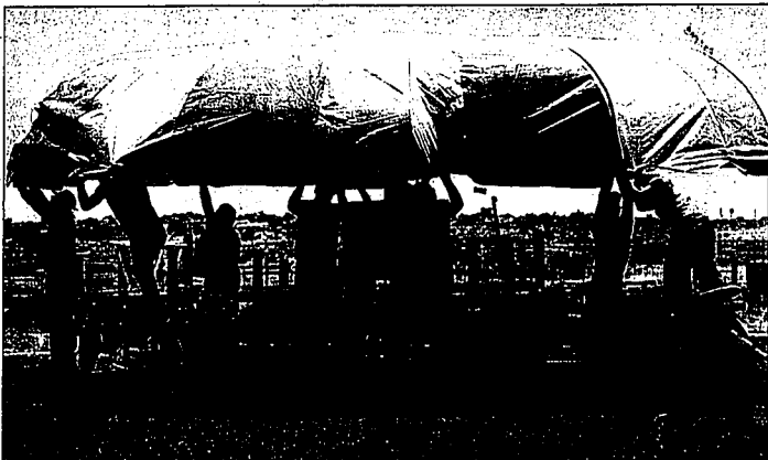
It takes plenty of hands to install a ride canopy during a breezy Monday in Shoshone. Danny Brown's carnival will feature 10 rides and eight games along with other attractions at the Lincoln County Fairgrounds.
