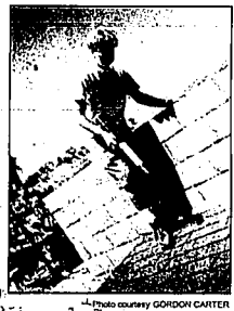
Daniel Brown of Murtaugh helps put a roof on an orphanage in Tijuana.
