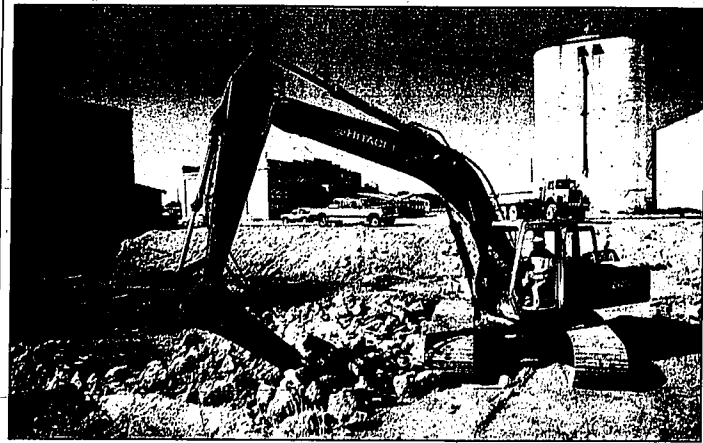
Don Johnston of Earth Rock Inc. uses a rock hammer on his excavator to break up concrete in a hole left from the Twin Falls Food and Ice building fire. The location may be transformed into a much-needed parking lot for Twin Falls' Old Towne area.
