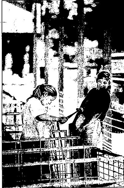
Mella McEwen, left, of Hazelton and Darla Cridder of Eden team up to install 4-H signs inside the new swine barn on Friday.
