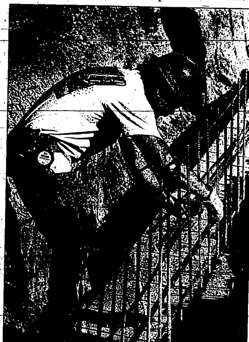
Rick Martinat secures re-bar at a construction site at the College of Southern Idaho. As Labor Day neared, working folk reflected on laborers' recent victories and defeats.
