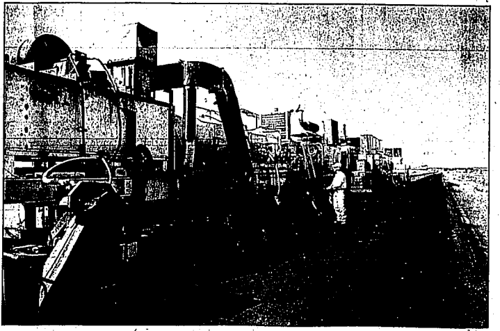
Robert Hanson, crew leader for Gordon Paving, works on an asphalt recycling train being used to repave a stretch of eastbound Interstate 84 near Burley Saturday. Hansen said the train removes old asphalt, heats it up, chews it up and lays it back down. A stretch of the interstate's westbound side is due to be completed in about two weeks.
