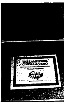
Hangar among photographs of movie stars, this sign tells passersby to expect a new cinema in Old Town - eventually. At left, Ruben Salazar of Twin Falls helps strip the foundation of Twin Cinema for remodeling.
