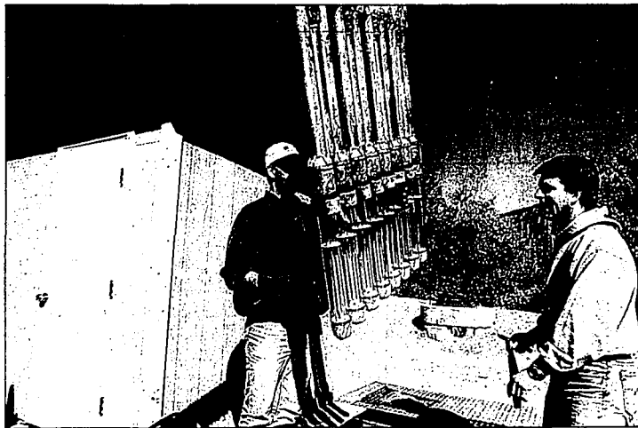
Richard Harrison, left, and Mike Sarchese check over the new ultraviolet light system at the Twin Falls sewage treatment plant. Harrison and Sarchese work for Trojan Technologies, Inc., a Canadian firm based in London, Ontario.
