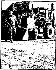
JOHN FLOER OF HOFFBAHR EXCAVATING CO. BREAKS GROUND IN SOUTH BURLEY TUESDAY EVENING FOR EXCAVATION.
