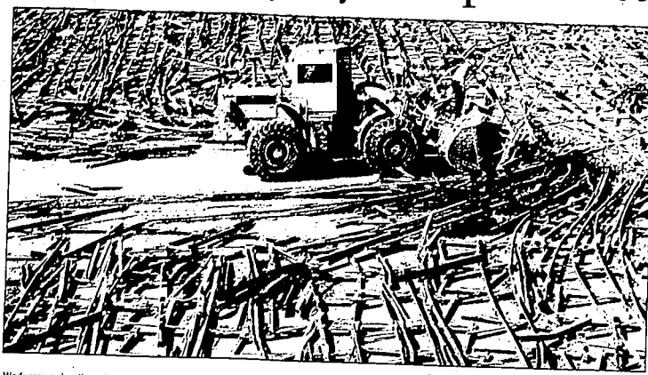
Work crews plow through what used to be acres of chicken coops at Egg City in Moorpark, Calif., last week. Egg City once had millions of chickens and was the largest employer in Moorpark, but closed this summer.
