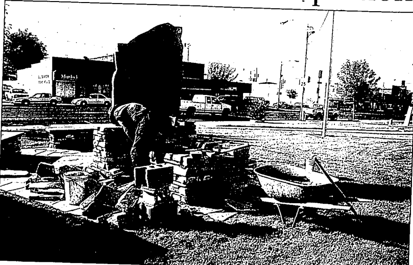
Albion stonemason Kent Hale works to complete an addition to the Veteran's Memorial at the Cassia County Courthouse.
