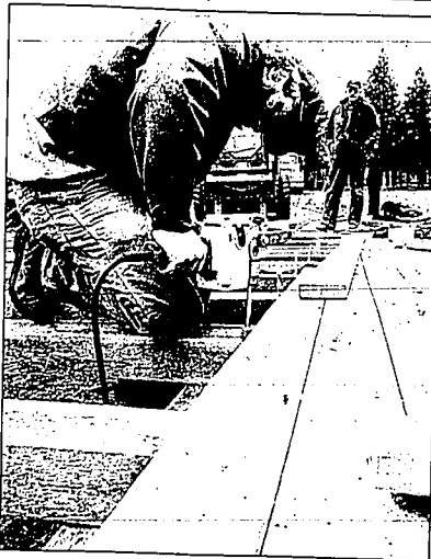
Yellowstone National Park maintenance worker Jim Heber drives a huge log screw into the foundation lumber of a new boardwalk at the viewing area of Old Faithful. The surface planks are not wood but plastic lumber, made from recycled detergent bottles and milk jugs.
