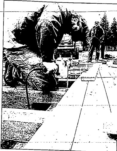
Yellowstone National Park maintenance worker Jim Haber drives a huge log screw into the foundation lumber of a new boardwalk at the viewing area of Old Faithful. The surface planks are not wood but plastic lumber, made from recycled detergent bottles and milk jugs.
