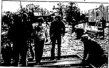
Gayle Purdy (center front), Ken Hill (left standing) and Weston Gray (kneeling on the right) are among the volunteers helping to construct Habitat for Humanity's third house in Twin Falls.
