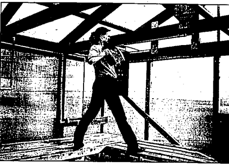
Amber Lafferty installs plumbing for the watering system inside the Bliss School greenhouse.
