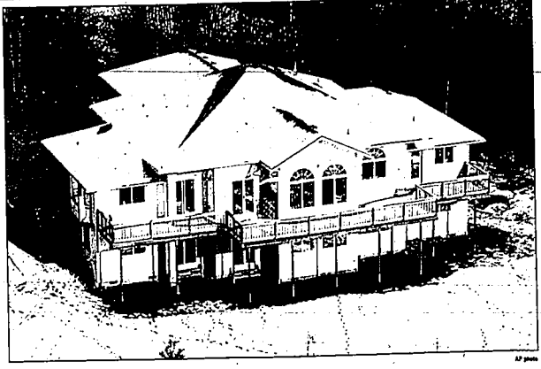
This 5,300-square-foot home on the Tulalip Indian Reservation near Seattle was built with taxpayer money earmarked for low-income housing. This house is owned by the chief administrator of the tribal housing authority and her husband, the agency's contracting officer.
