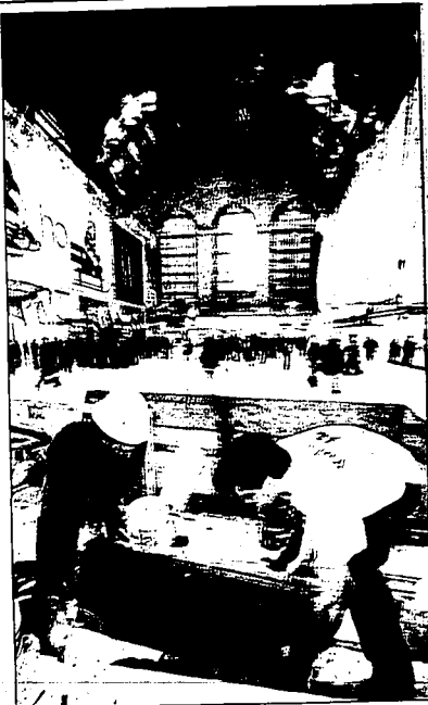
Stonemasons lay a section of marble during the restoration of the grand staircase in New York's Grand Central Terminal on Tuesday. The terminal is undergoing a $175 million restoration.
