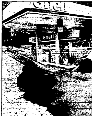
Police officers look over a sinkhole that opened under a Shell gas station in Lake Forest Park, Wash., Wednesday. Parts of the station sank six to eight feet after a heavy storm hit the Northwest.
