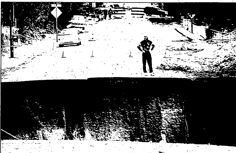
A jogger comes to a hole he can't jump as he views a 30-by-100-foot sinkhole that swallowed a three-way intersection in Shoreline, Wash., Wednesday. The combination of snow melt, rain, broken water and drainage lines contributed to the washout.
