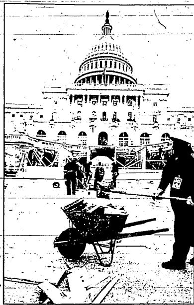
Work continues on Capital Hill Thursday for the Presidential Inauguration stand. President Clinton will be sworn in for his second term Jan. 20.
