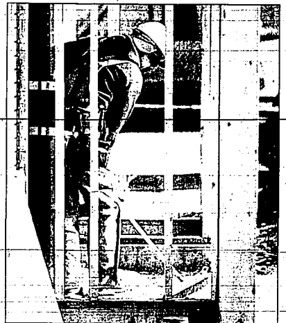
Tom Owens cleans up while working on the remodeling of the building site of the new D.L. Evans Bank on Main Avenue in Twin Falls.
