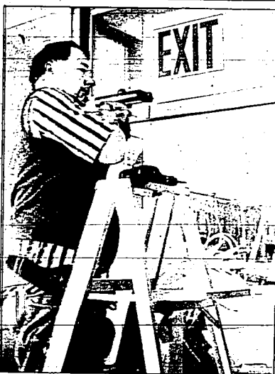
Don Walters works Friday installing new hardware on a door at the Drift Inn. The business has been given notice that it doesn't meet state fire codes due to some minor violations.
