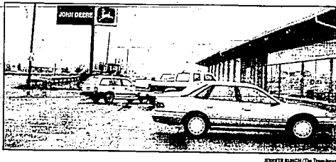
Expanding Overland Avenue from two lanes to four to accommodate bridge construction would move the road east and nearly to the rear of the vehicles parked here in front of Christiansen Implement in north Burley.
