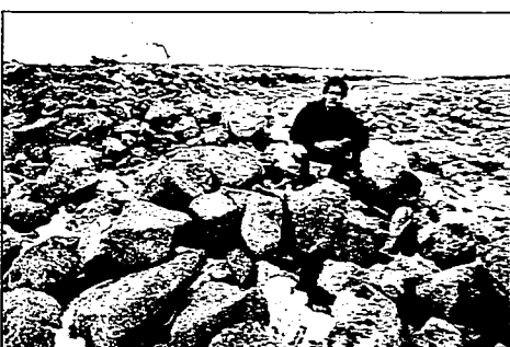
Twin Falls water superintendent Mike Trabert shows where an old "rock check" had existed in the Low-line Canal. It could be built back into a small dam in an effort to recharge some of the city's water supply.
