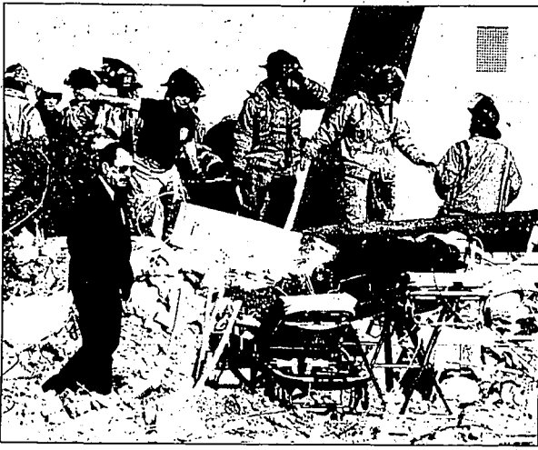
Houston firefighters carry an unidentified injured person from the scene of a collapsing wall at a Houston mall Thursday. The collapse killed two and injured at least six.
