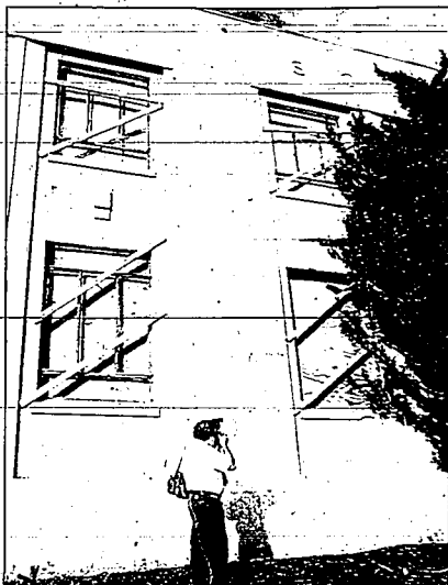
Roberto Padilla, with the Salano County Public Defender's Office, photographs the exterior wall of the Salano County Courthouse, in Vallejo, Calif., where a bomb exploded Thursday. Two suspects are in custody.
