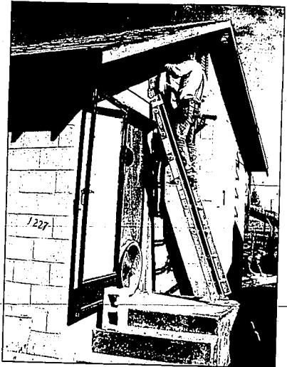
Carpenters Ed Campos, left, and Randy Wright, of the South Central Community Action Agency weatherization program, work to make a Burley home more energy efficient. The orange device covering the front door is used to change pressure inside the home and pinpoint areas where warm air escapes outside.
