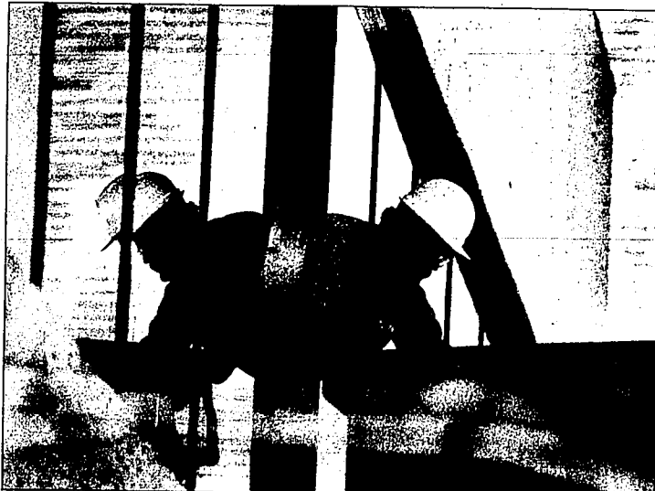
Taking the trash out appears to be double duty for a construction worker at the College of Southern Idaho. Several days of gutting the old library on the second floor of the Taylor administration building has prepared the way for new offices as part of the remodeling project.
