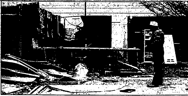
Franklin Dunn surveys damage to a neighbor's house Friday after a tornado touched down north of Lubbock, Texas, Thursday night. The frame structure was destroyed by one of several twisters in the area that resulted in at least one death. Dunn's home, three miles north of this house, was not damaged by the storm.
