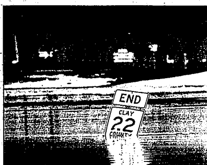
The county highway ends in the floodwaters of the Red River on the border of Minnesota and North Dakota in Moorhead, Minn., Sunday.
