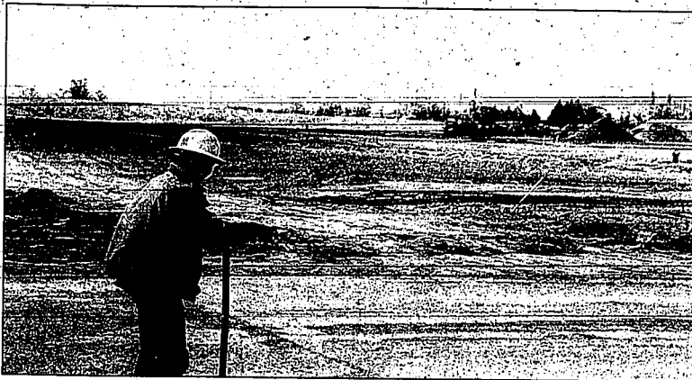
Randy Williams, an employee of R&S Construction Co., Rexburg, charges water lines Thursday afternoon at the site of the new Burley High School building. JOE PETERSON/The Times-News
