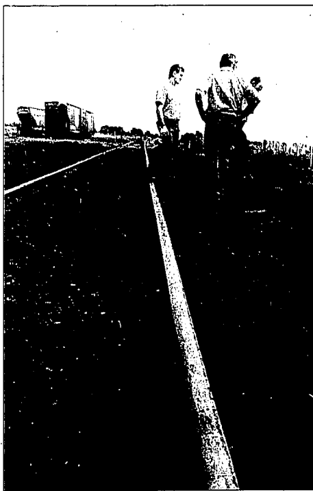
Mike Pfeigler, left, of the Idaho Transportation Department, surveys the railroad tracks crossing Idaho Highway 25 just west of downtown Jerome. The highway will be closed for 30 days while work crews from Eastern Idaho Railroad repair the intersection.
