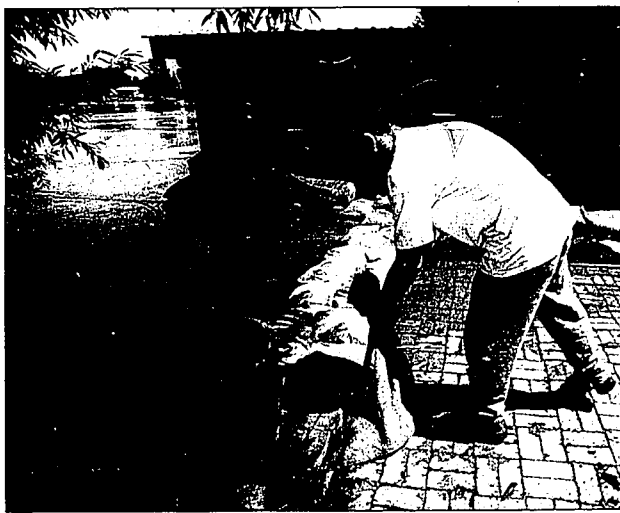
Volunteer Chris Welch of Buhl plants an additional sandbag Friday on a growing pile that is meant to prevent water from entering a house on Bell Rapids Road in Hagerman. Sandbag lines increased in number near houses along the riverside as water levels continued to rise.
