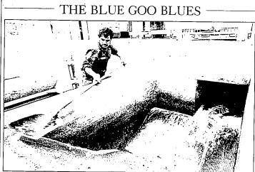
Mario Estrada cloans out the screen where water and sludge from washing denim drain out of international Garment Processors' laundry department. The El Paso, Texas, firm is researching dumping the sludge on farmiand to boost crop production.
