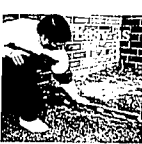
1. Excavate and prepare the base. Dig a shallow trench, then compact and level the soil.
