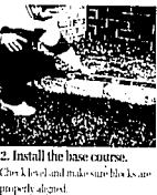
2. Install the base course. Check level and make sure blocks are properly aligned.
